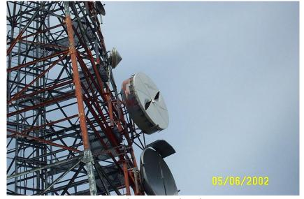
**Figure 3: Heavily Damaged Radome**
