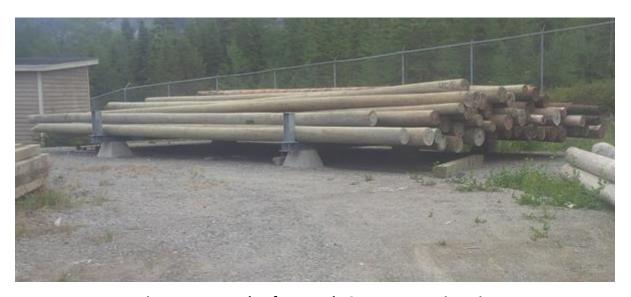
Figure 1: Example of New Pole Storage Ramp in Nain
