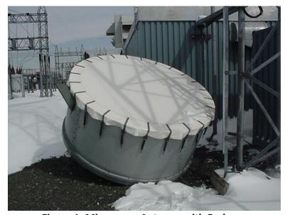
Figure 1: Microwave Antenna with Radome
