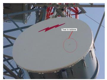
Figure 2: Tear in Radome
