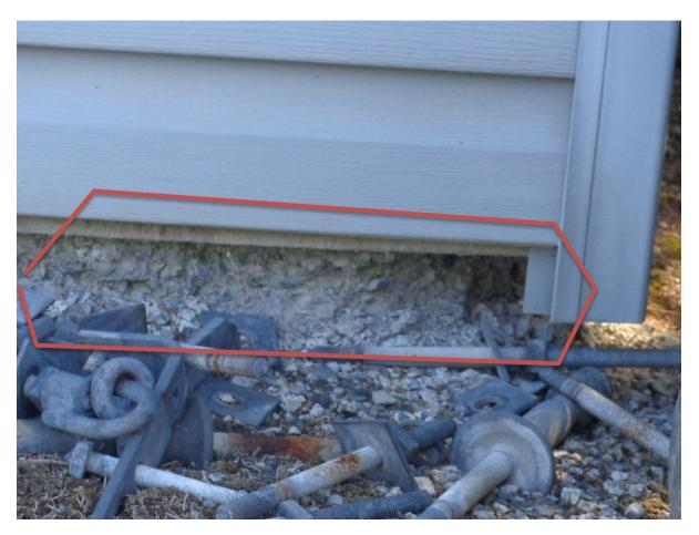
Figure 4: Deteriorated Concrete Slab under the Storage Shed walls
